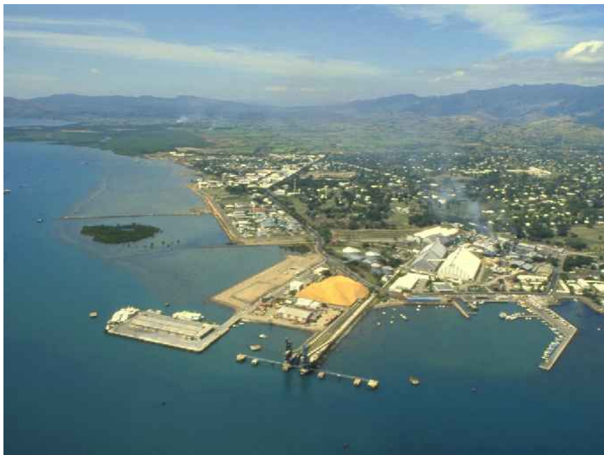
Lautoka wharf area from the west
